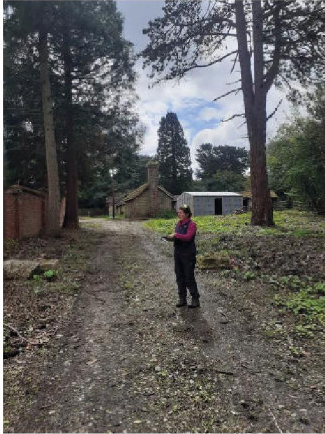
Photograph 1: View into the site from the entrance at the end of Dukes Hill showing the existing buildings.
